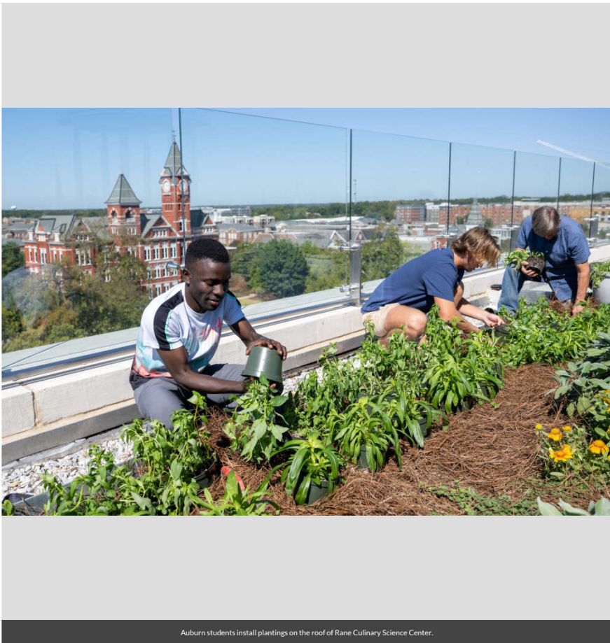
Auburn students install plantings on the roof of Rane Culinary Science Center.
