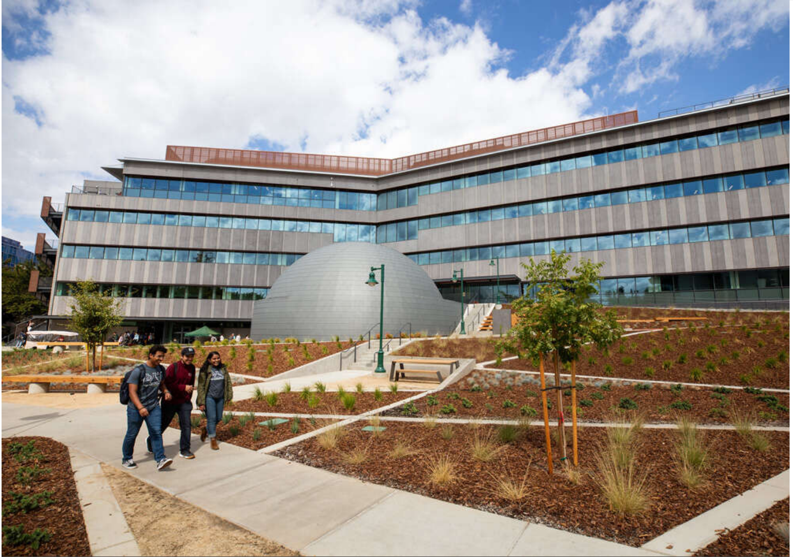
Tschannen Science Complex has an integrated living roof that provides thermal barriers for the building as well as being home to a refuge for pollinators and a native plant garden
