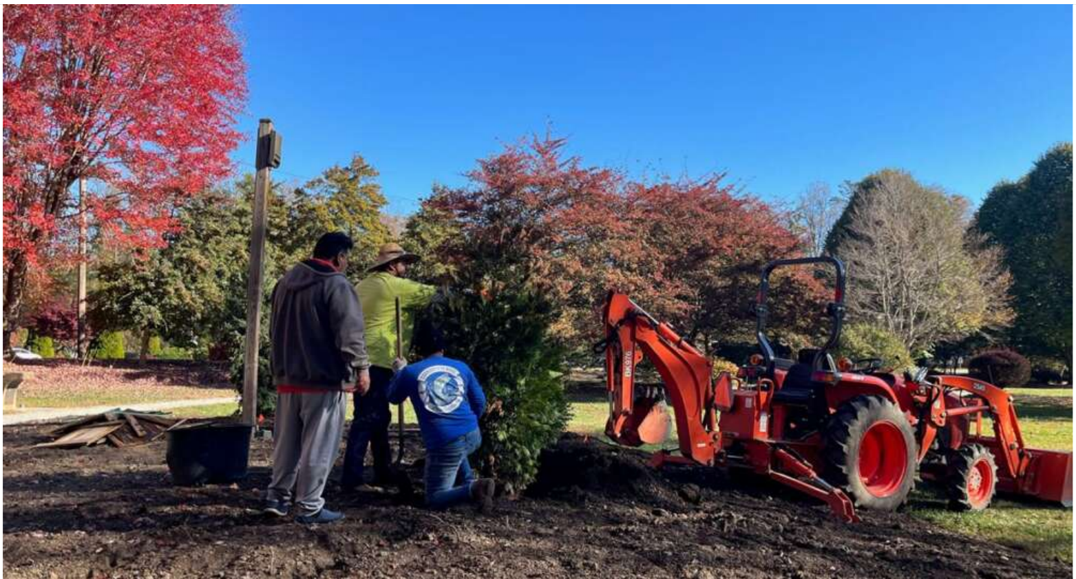
Installation of the Christmas tree bed during the first installment of plants in Laurel Green on October 24, 2022
