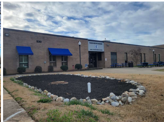
The second rain garden is located in a low-lying area at the Early College High School, located at the back of NCC's campus. The low grassy area has a drain in the middle, so it feeds into the underground network of storm drains. It catches runoff and sediment from the parking lot, so this prevents standing water on the parking lot and sidewalk.
