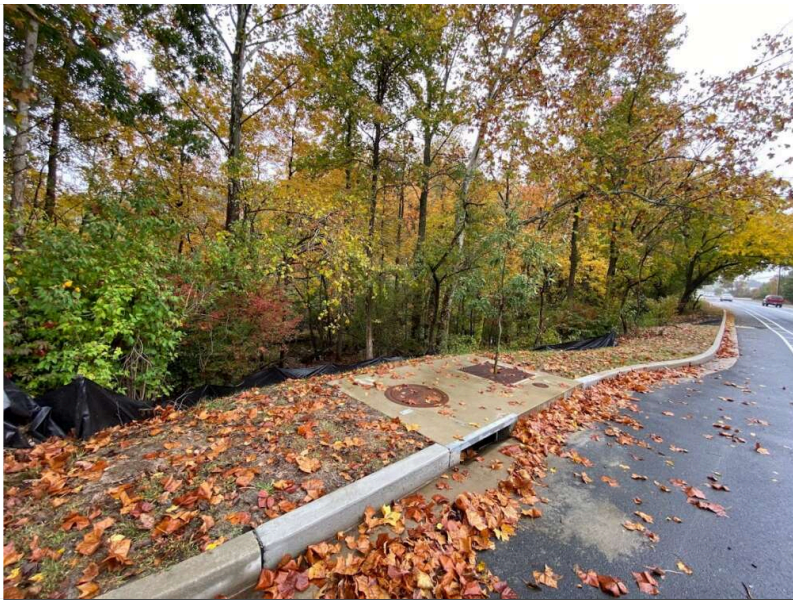
Pictured is what looks like a typical stormwater runoff drain but is instead a filterra system which uses biologic processes to collect the nutrient runoff into the soil, this enhances the surrounding system which has many native shrubs and pollinator friendly trees.
