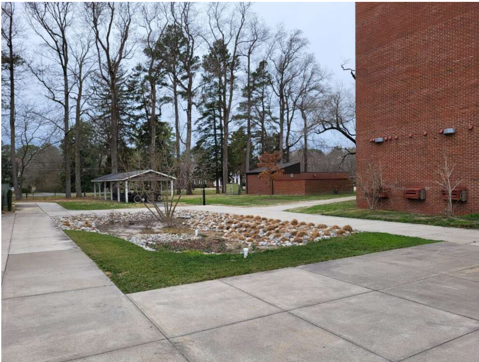
Native Bioswale located adjacent to Choptank Hall.
