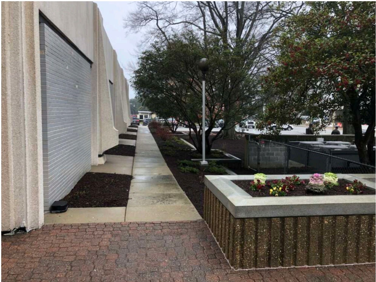
Just one side of City Hall Complex City Maintain IPM standard Photo Credit: David S. Freeman
