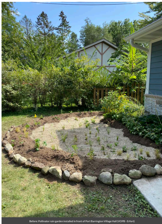
Before: Pollinator rain garden installed in front of Port Barrington Village Hall (VOPB - Erfort)
