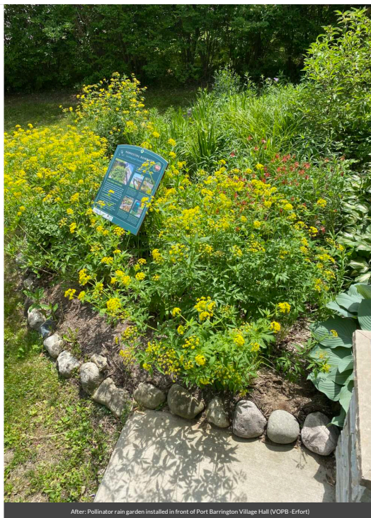
After: Pollinator rain garden installed in front of Port Barrington Village Hall (VOPB - Erfort)
