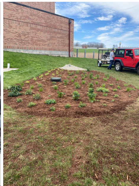
Setting up the rain garden at the UConn Dairy Bar (photo credit: Amanda Stowe)
